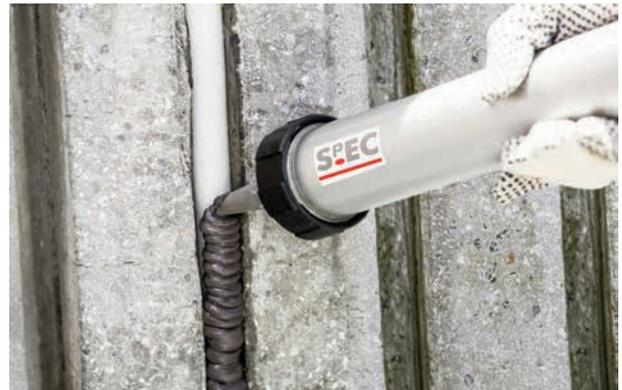
The joint faces should be protected with masking tape to facilitate tooling.
